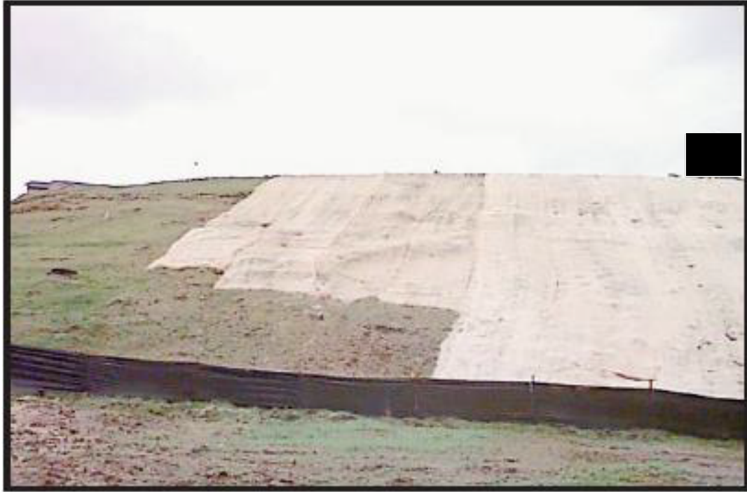
Plate 3 – Coconut matting and silt fence (Source: CIRIA, 2006 10 )
