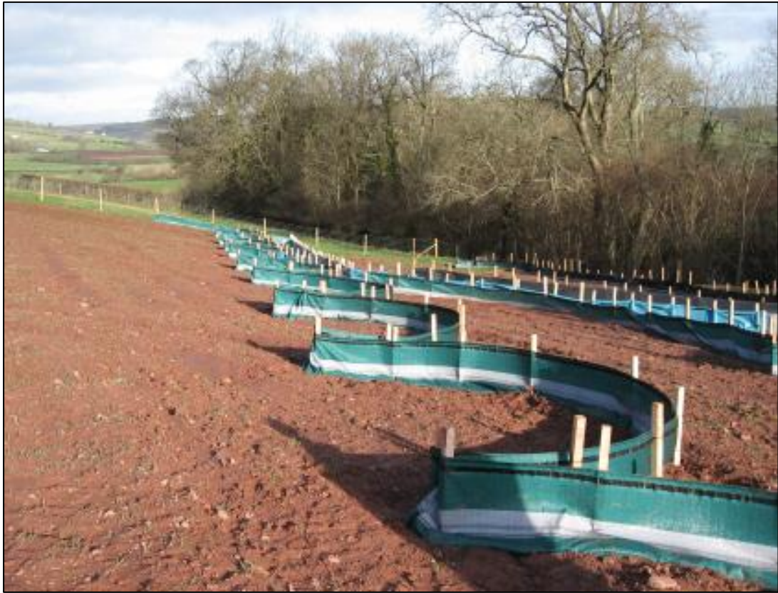
Plate 2 – Example of good practice in silt fence installation (Source: Geosynthetics, 2021 12 )
